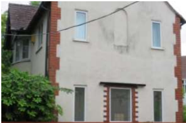
Side (west) elevation of no.79 Austin Drive
